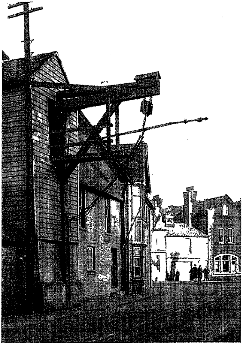
Cart Weighing Steelyard in Soham, Cambridgeshire
